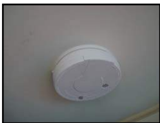
Figure 2-7. Smoke Detector
