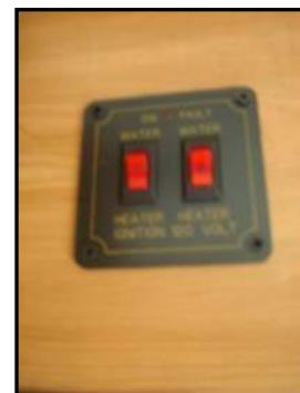
Figure 4-15. Water Heater Switches
