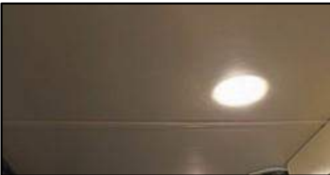
Figure 12-3: Typical Ceiling in the Allegro Breeze
