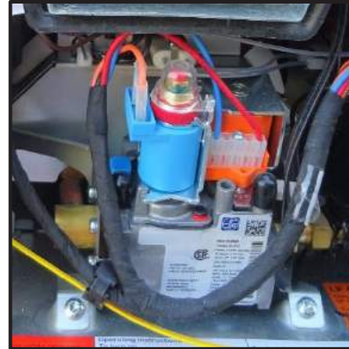
Figure 5-10: Water Heater Relief Valve
