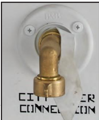
Figure 13-7: City Water Supply Connection
