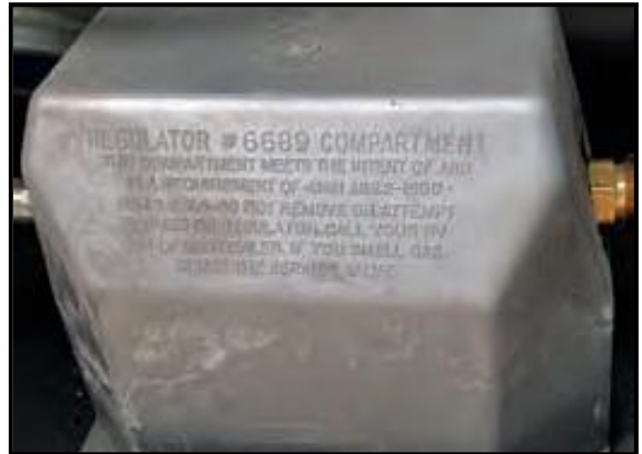
Figure 4-2: LP Gas Regulator
