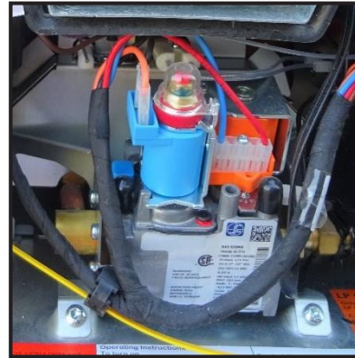
Figure 5-10: Water Heater Relief Valve
