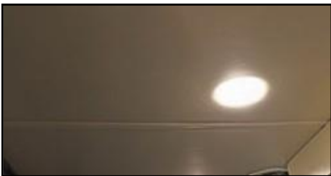
Figure 12-3: Typical Ceiling in the Allegro Breeze
