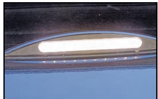
Figure 11-3: Exterior Security Light
