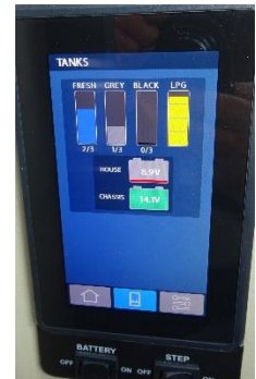
SPYDER Control showing approximate amount of LP Gas Remaining in Tank.
