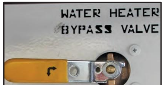
Figure 13-9: Water Heater Bypass System
