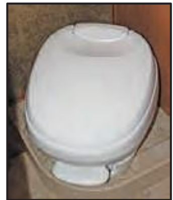
Figure 13-10: Toilet Pedal Flush Lever
