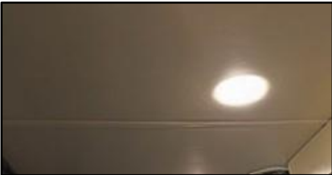
Figure 12-3: Typical Ceiling in the Allegro Breeze
