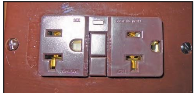
Figure 9-12: GFCI Receptacle
