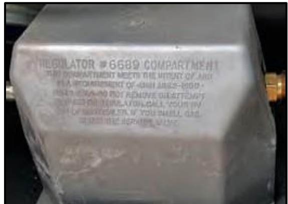
Figure 4-2: LP Gas Regulator
