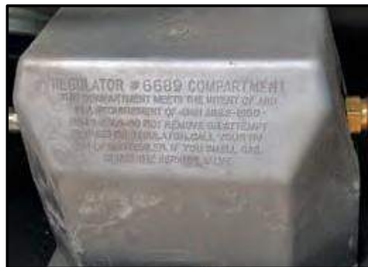
Figure 2-4: LP Gas Regulator
