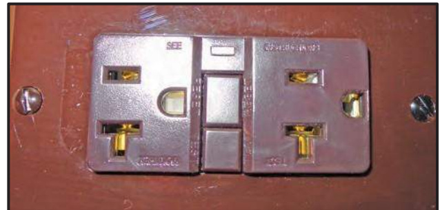
Figure 9-11: GFCI Receptacle
