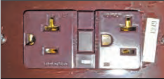
Figure 9-10: GFCI receptacle
