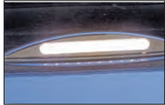
Figure 11-3: Exterior security light
