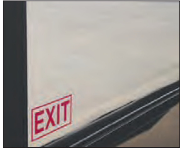
Figure 2-9: Emergency exit window
