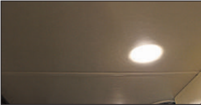
Figure 12-3: Typical ceiling in the Allegro Breeze
