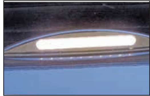
Figure 11-3: Exterior security light
