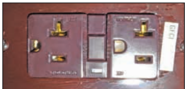
Figure 9-8: GFCI receptacle
