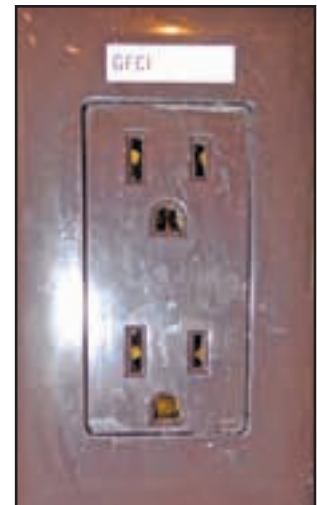
Figure 9-5: 120 VAC receptacle
