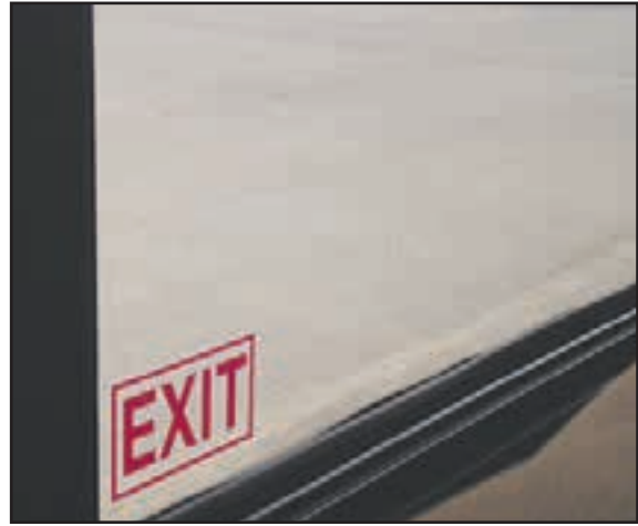
Figure 2-9: Emergency exit window
