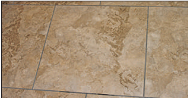
Figure 12-2: Typical flooring in the Allegro Breeze
