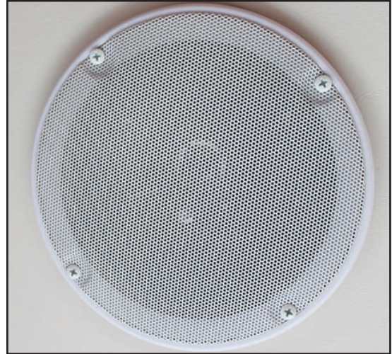
Figure 6-3: Overhead surround sound speaker
