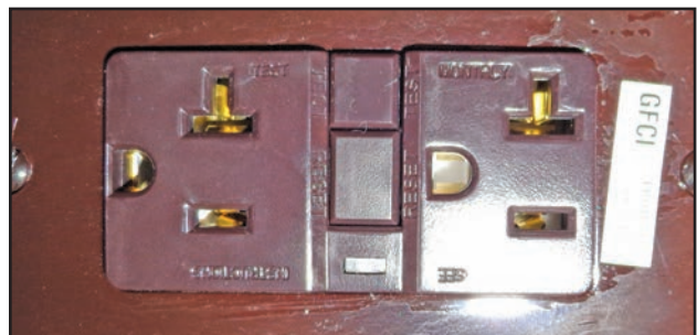
Figure 9-8: GFCI receptacle
