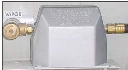
Figure 3-5. LP Gas Regulator
