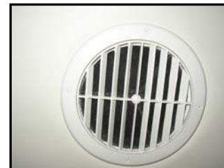
Figure 3-2. Round Vent/Filter
