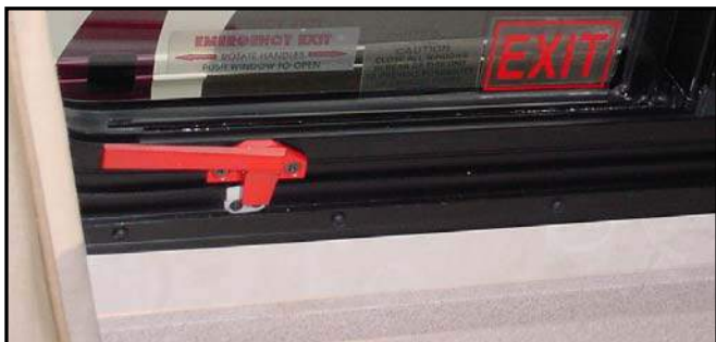
Figure 12-2. Bedroom Emergency Exit Window
