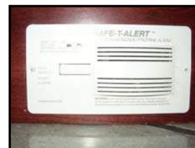
Figure 4-15. Carbon Monoxide/LP Gas Detector
