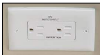
Figure 7-7. GFCI Receptacle
