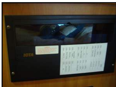
Figure 7-1. Circuit Breaker Box
