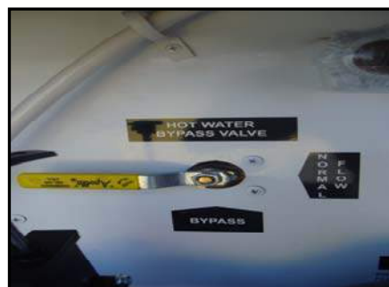
Figure 11-9. Water Heater Bypass System
