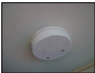
Figure 2-7. Smoke Detector
