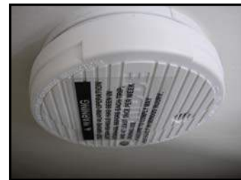
Figure 13-19. Smoke Detector
