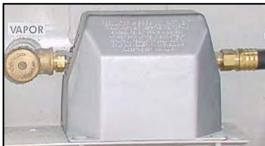
Figure 3-5. LP Gas Regulator
