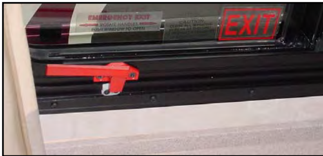
Figure 12-2. Bedroom Emergency Exit Window
