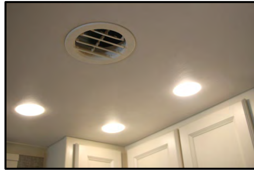
Figure 3-3: Outgoing Air Vents
