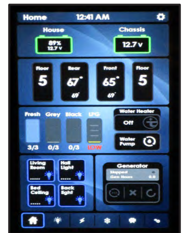
Figure 9-4 Multiplex System Switch Panel
