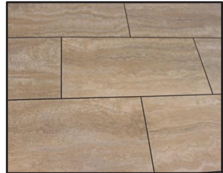
Figure 12-2: Typical Flooring in the Allegro Bay
