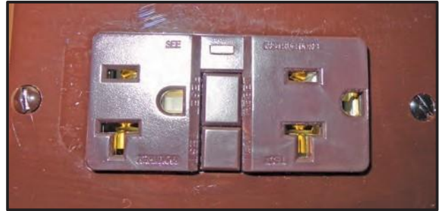
Figure 9-5: GFCI Receptacle
