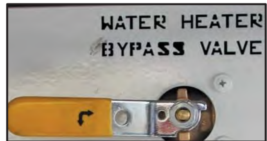
Figure 13-9: Water Heater Bypass System
