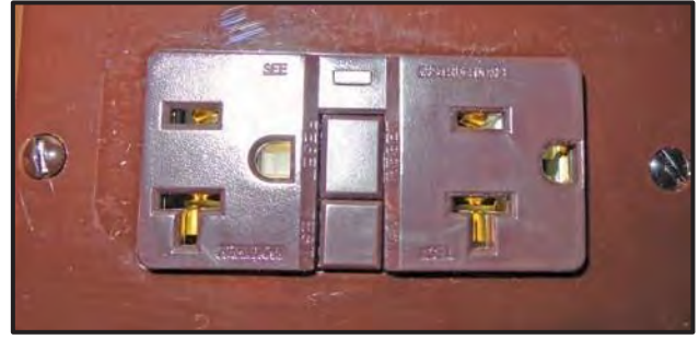
Figure 9-5: GFCI Receptacle
