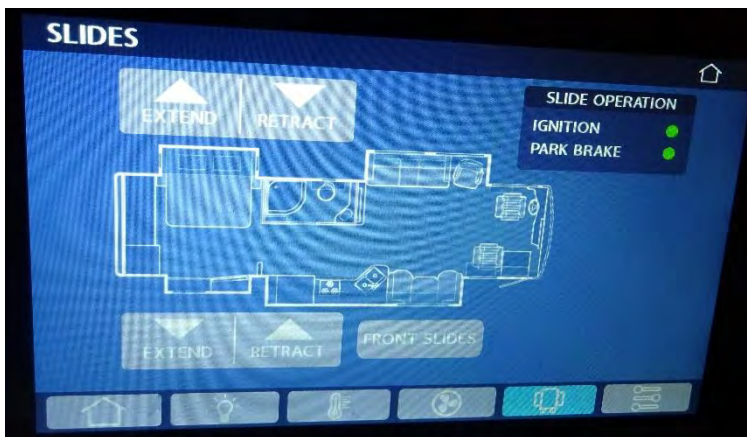
Figure 10-1: Slide-Out Screen on the Spyder Controls System
