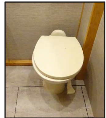
Figure 13-10: Toilet Pedal Flush Lever
