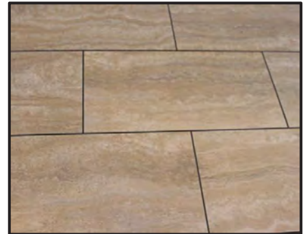
Figure 12-2: Typical Flooring in the Allegro Bay
