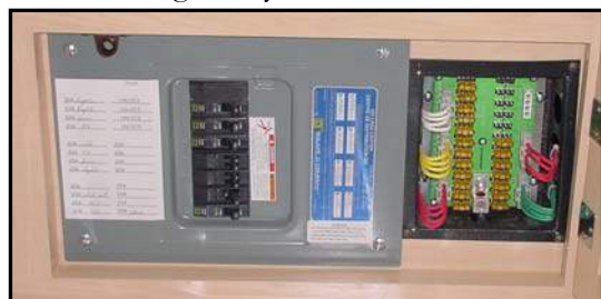
Figure 7-1. Circuit-Breaker Box
