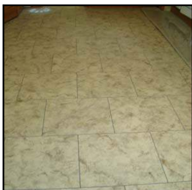
Figure 10-2. Typical Flooring (Carpeting and Tile)
