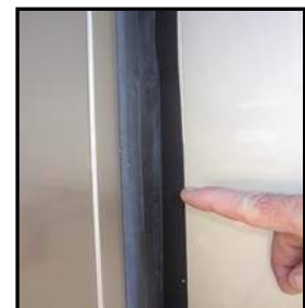
Figure 14-5. Inspecting Slide Out Gasket
