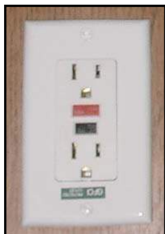
Figure 7-7. GFCI Receptacle
