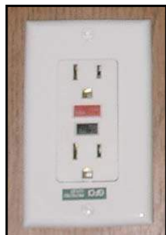
Figure 7-7. GFCI Receptacle
