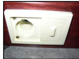
Figure 14-9. Vacuum Hose Coupling
