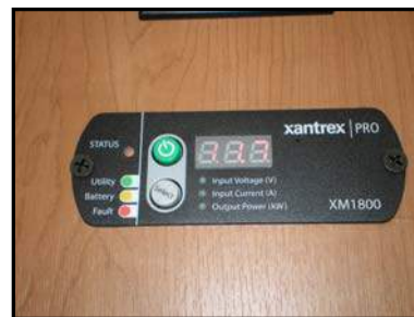
Figure 7-10. Inverter Control Panel
