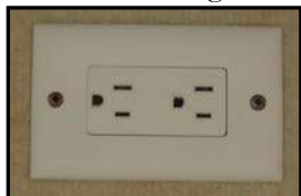
Figure 7-5. 120 VAC Receptacle
