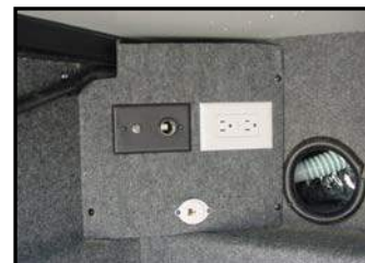
Figure 4-15. Cable & Telephone Jack
