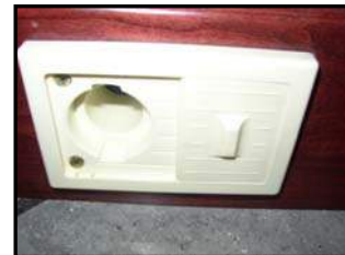
Figure 14-9. Vacuum Hose Coupling
