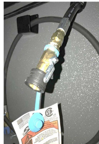
Figure 4-5: LP Quick Connect Lever On Position
