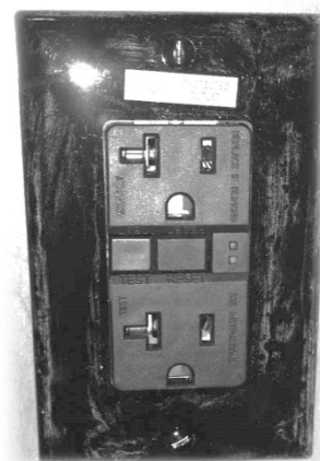
Figure 9-7: GFCI Receptacle
