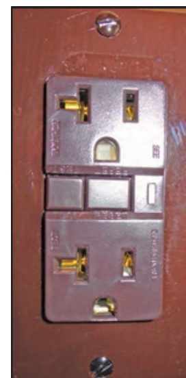
Fig. 9-5: GFCI Receptacle
