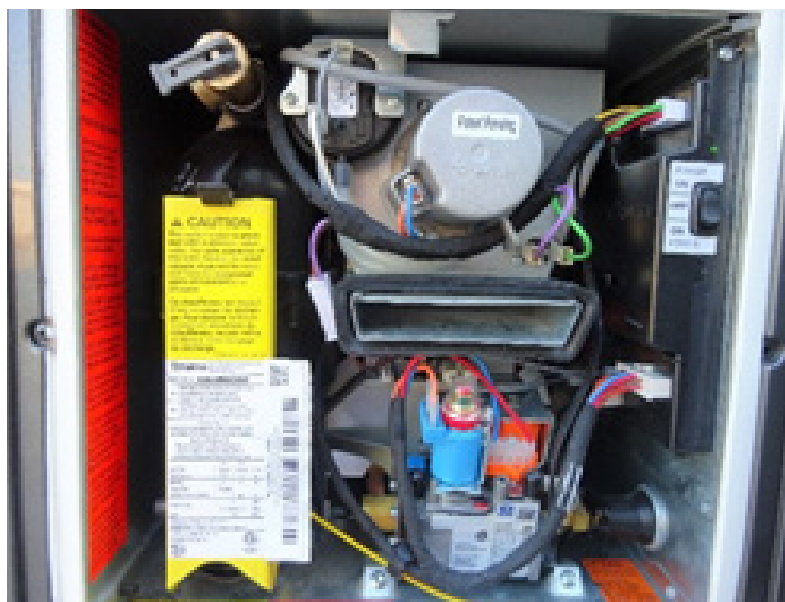
Fig. 5-8: Tankless Water Heater
