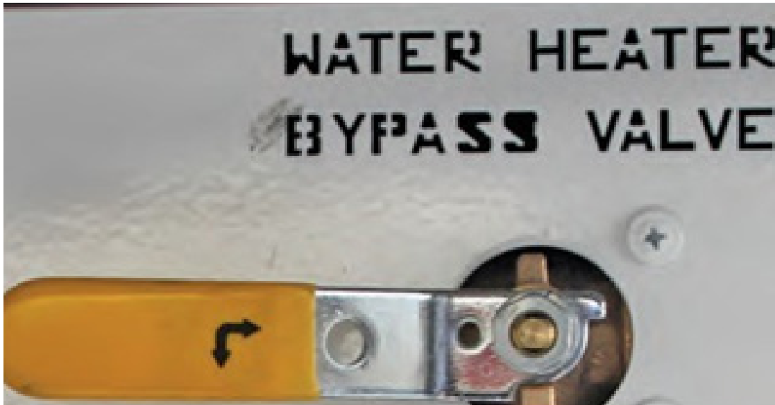
Fig. 13-10: Water Heater Bypass
