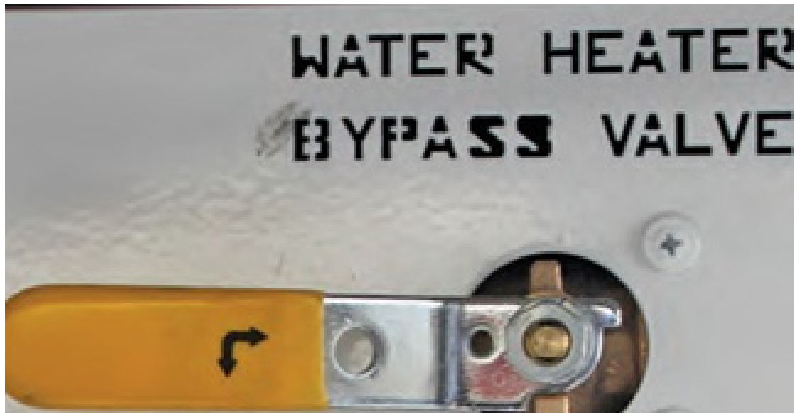
Fig. 13-10: Water Heater Bypass
