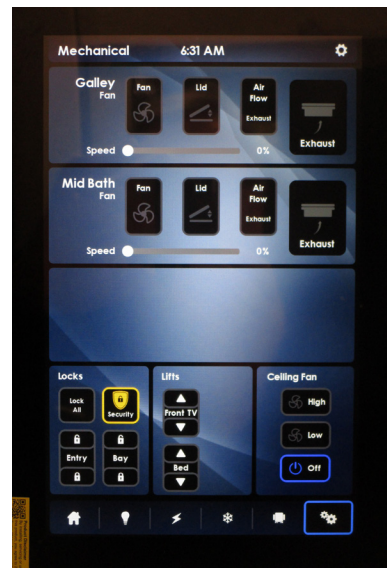
Fig. 6-3: Spyder Television Lift Control
