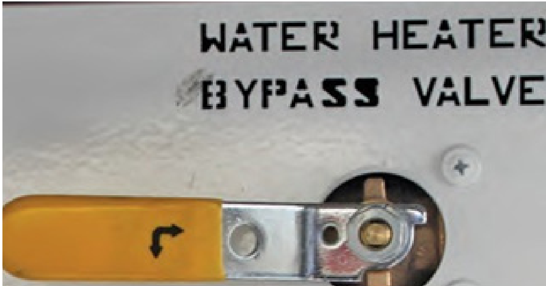
Fig. 13-10: Water Heater Bypass
