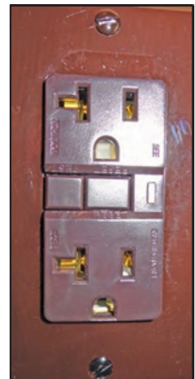
Fig. 9-5: GFCI Receptacle
