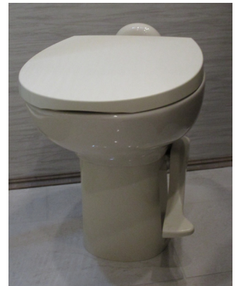
Fig. 13-12: Toilet with Pedal Flush Lever
