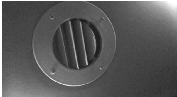
Figure 3-2: Round Air Vent
