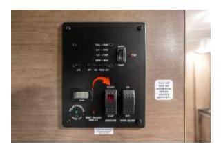
Image 63.2 Generator Start/Stop Button On Control Panel
