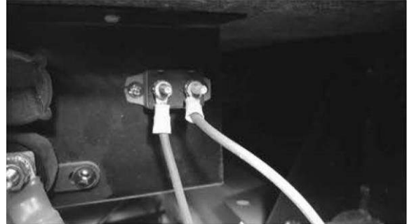
Figure 10-1: Equalizer Fuse Block
