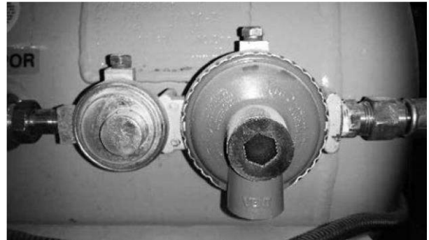
Figure 2-4 LP Gas Regulator
