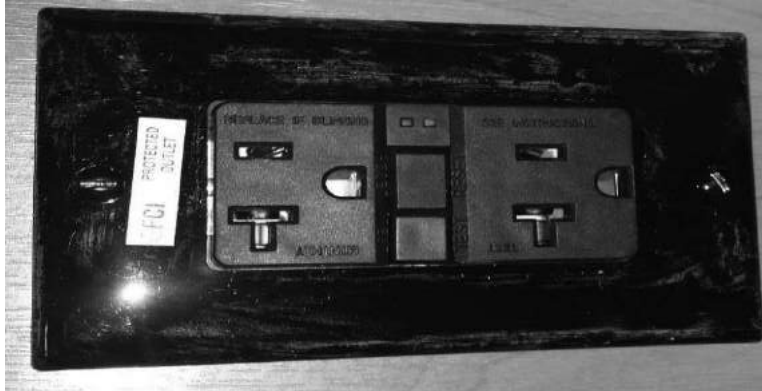
Figure 9-5 GFCI Receptacle
