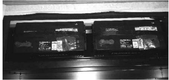
Figure 9-2: House Batteries
