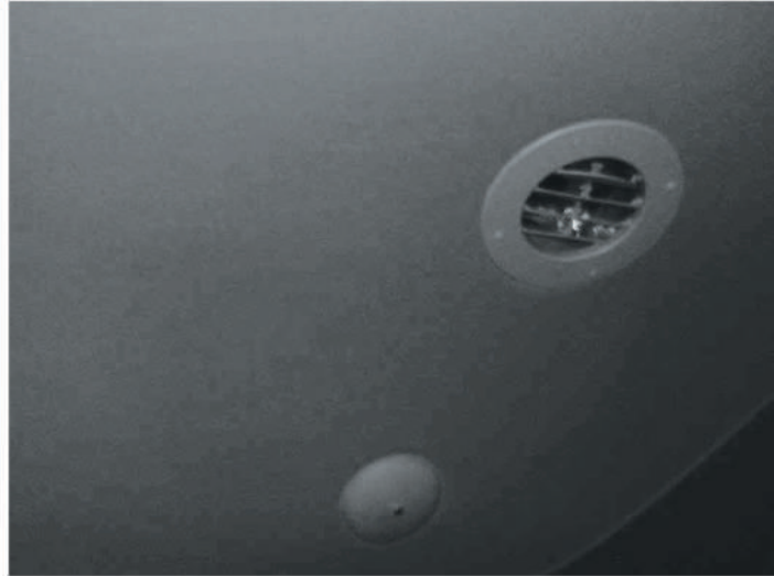
Figure 12-3: Typical ceiling in the Wayfarer
