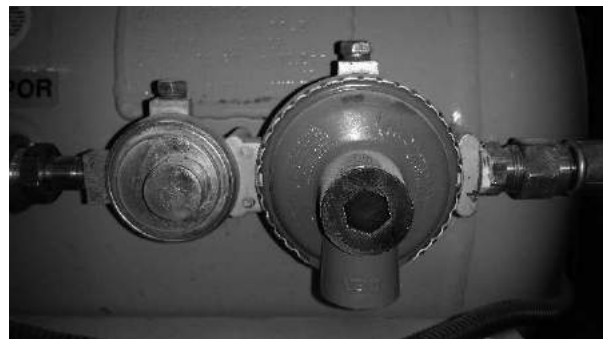
Figure 2-4 LP Gas Regulator
