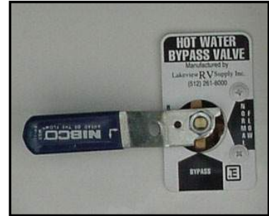
Figure 11-7. Water Heater Bypass Valve
