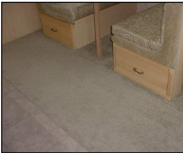
Figure 10-2. Typical Flooring (Carpeting and Tile)
