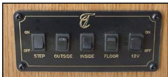
Figure 7-4. Battery Disconnect Panel
