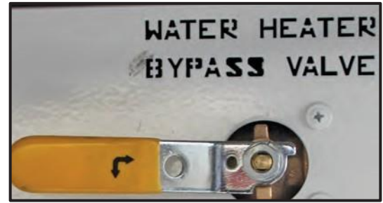
Figure 14-10: Water Heater Bypass System
