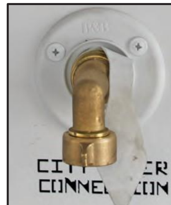
Figure 14-8: City Water Supply Connection
