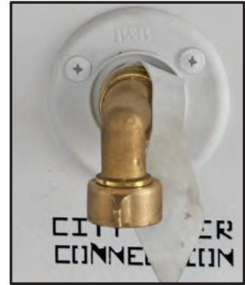
Figure 13-7: City Water Supply Connection
