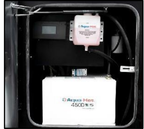
Figure 13-18: Aqua-Hot Surge Tank
