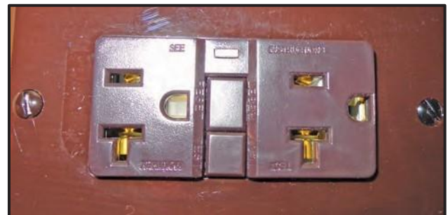
Figure 9-9: GFCI Receptacle
