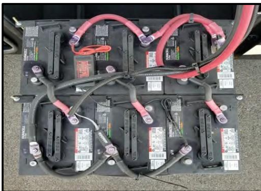
Figure 9-3: House Batteries
