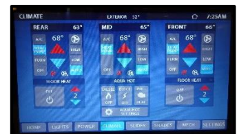
Figure 4-7: Heat Pump Controls
