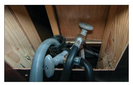
Figure 86. Washing Machine Shutoff Valves
