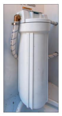
Figure 58. Water Filter Housing
