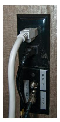
**Figure 99.** Cable/Satellite Outlet—Bedroom
