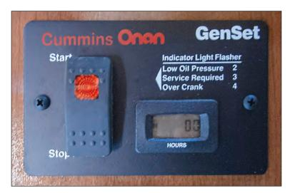
Figure 28. Generator Control Panel
