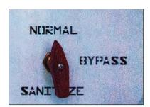
Figure 55. Water Heater Bypass Valve
