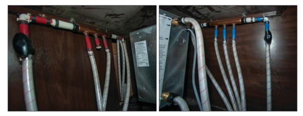
Figure 43. Hot and Cold Water Shutoff Valves Behind Water Heater
