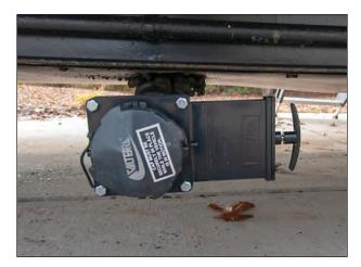
Figure 65. Sewer Outlet Connection (Termination Valve)
