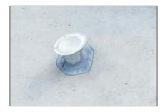
Figure 63. Roof Vent
