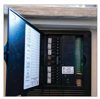
Figure 30. 12V Fuse Panel
