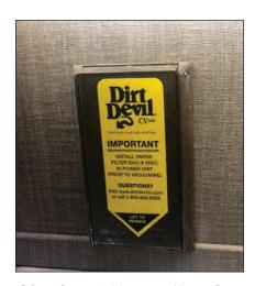
Figure 90. Central Vacuum Hose Connection
