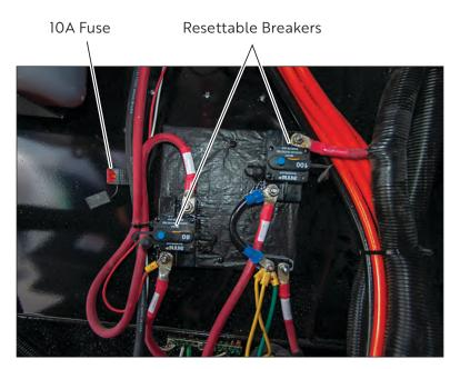
Figure 141. 10A Fuse and Resettable Breakers for Jacks/Leveling System
