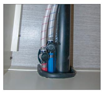
**Figure 52.** Bathroom Sink Shutoff Valves
