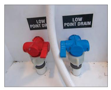
**Figure 55.** Low-Point Drains (Located in the Wet Bay)
