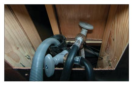
Figure 87. Washing Machine Shutoff Valves
