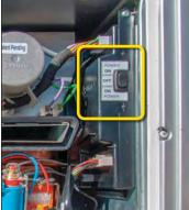
Figure 74. Truma Water Heater Control Dial and On/Off Switch
