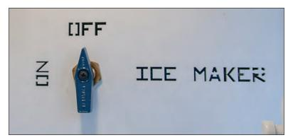
Figure 72. Ice Maker Valve in Wet Bay
