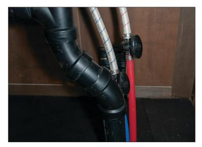
Figure 53. Kitchen Sink Shutoff Valves
