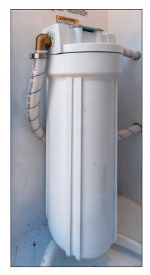
Figure 59. Water Filter Housing
