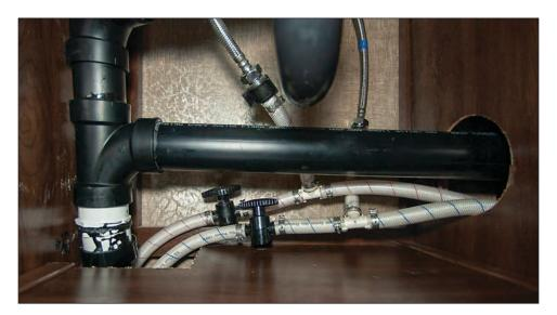
Figure 51. Bathroom Sink Shutoff Valves
