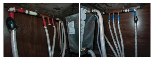
Figure 44. Hot and Cold Water Shutoff Valves Behind Water Heater
