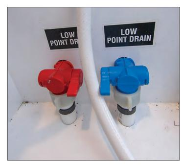
Figure 69. Low-Point Drains located under the RV
