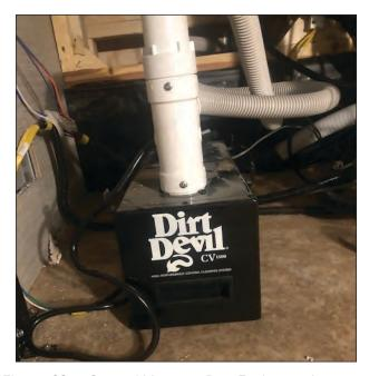
Figure 92. Central Vacuum Bag Exchange Location
