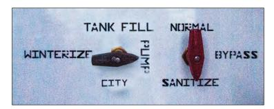
Figure 61. Sanitizing the Fresh Water System
