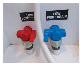
Figure 77. Low-Point Drains
