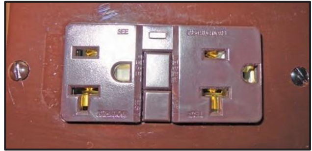
Figure 8-15: GFCI Receptacle
