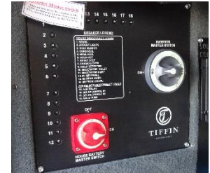
Figure 8-4: House Battery Disconnect Panel Switch
