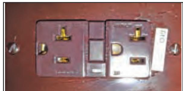
Figure 8-13: 120 VAC GFCI receptacle
