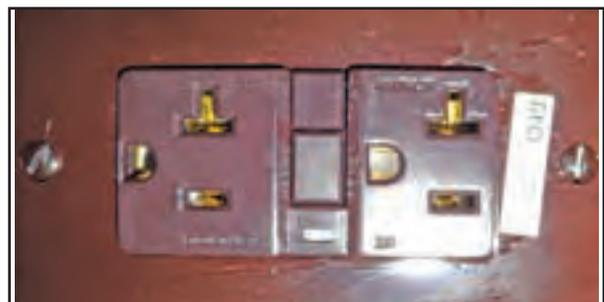
Figure 8-13: 120 VAC GFCI receptacle
