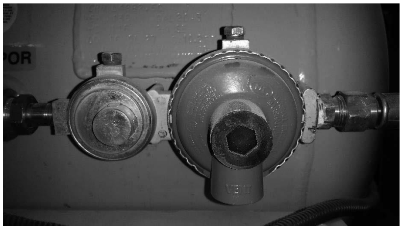
Figure 4-2: LP Gas Regulator
