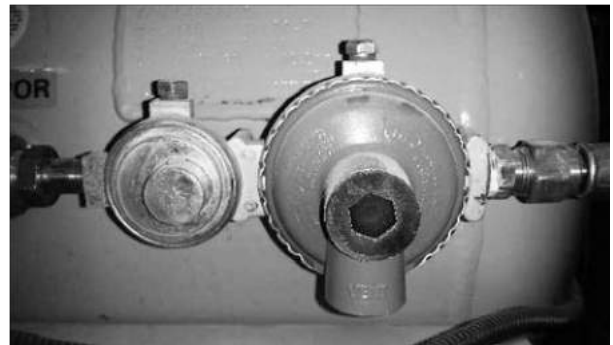
Figure 2-4 LP Gas Regulator
