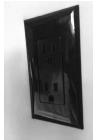
Figure 9-3:120 VAC Receptacle
