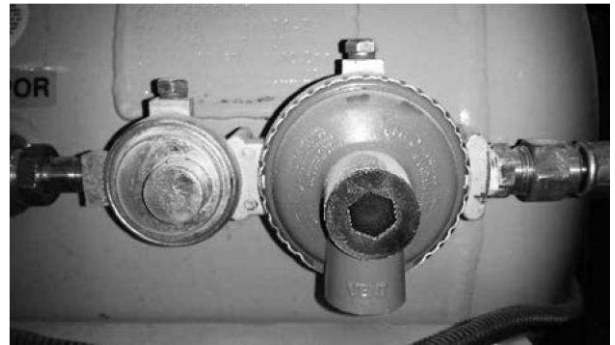
Figure 2-4 LP Gas Regulator
