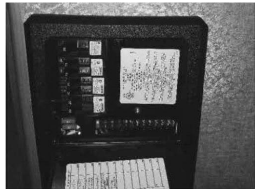
Figure 9-9: Main 120 VAC Load Center
