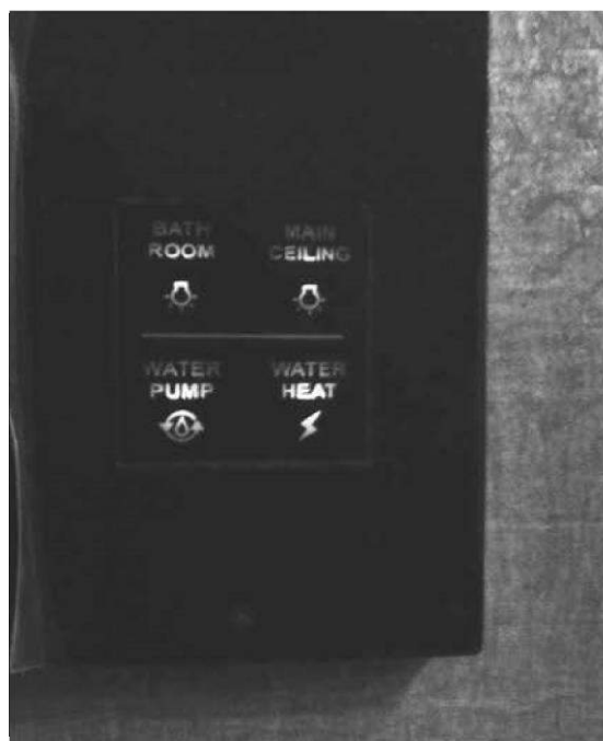
Figure 5-5: Water Heater Switch
