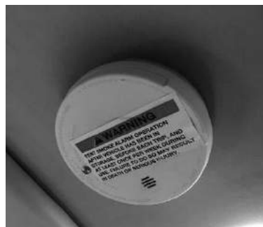
Figure 2-7: Smoke Detector
