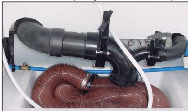
Figure 11-10. Sanitation Coupling, Valve, and Hose
