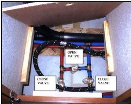
Figure 11-8. Water Heater Bypass System
