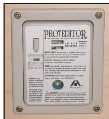
Figure 3-5. Propane Gas Detector
