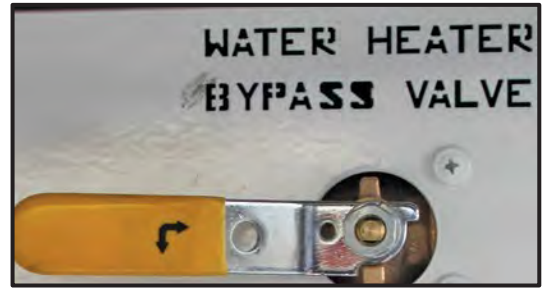
Figure 13-9: Water Heater Bypass System
