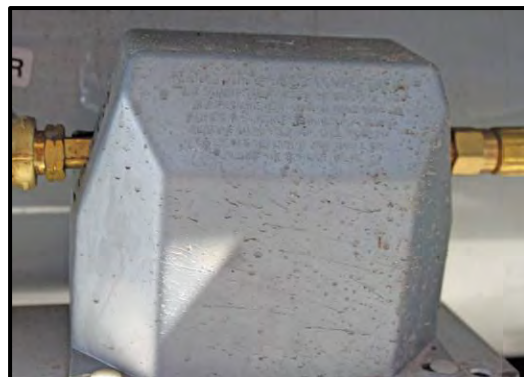
Figure 2-4: LP Gas Regulator
