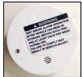
Figure 16-12: Smoke Detector
