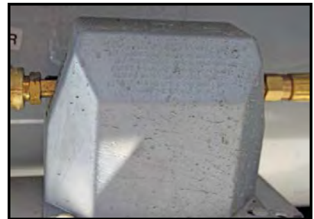
Figure 4-2: LP Gas Regulator
