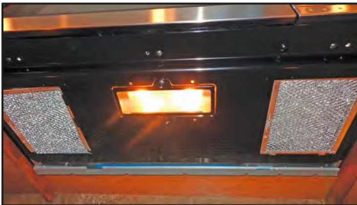
Figure 5-5: Air Filtration Fan
