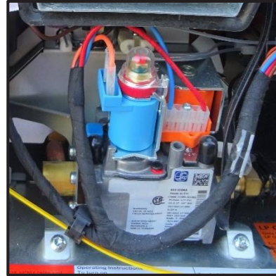
Figure 5-9: Water Heater Relief Valve
