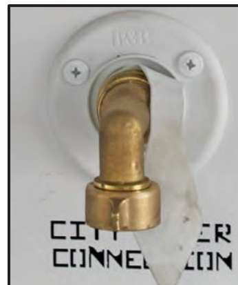
Figure 13-7: City Water Supply Connection
