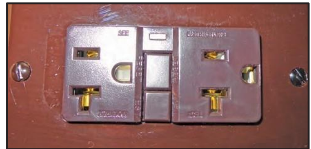
Figure 9-7: GFCI Receptacle
