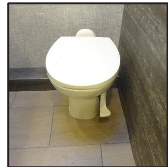
Figure 13-10: Toilet Pedal Flush Lever
