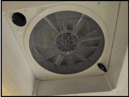
Figure 13-4: Overhead Vent Fan
