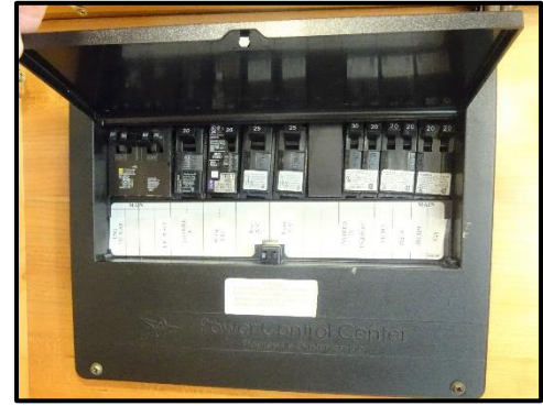
Figure 9-10: Circuit Breakers
