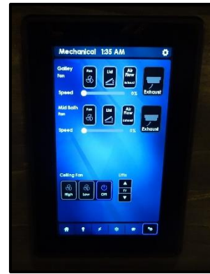
Figure 9-1: Spyder Controls System
