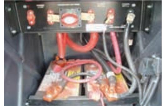
Figure 7-5. 12 VDC Battery System
