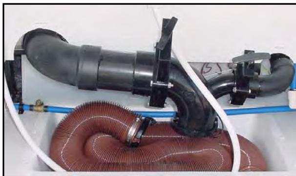
Figure 11-11. Sanitation Coupling, Valve, and Hose
