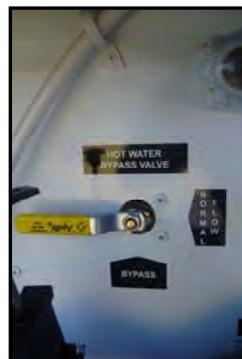
**Figure 11-9. Water Heater Bypass System**
