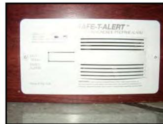
**Figure 3-6. CO/LP Gas Detector**
