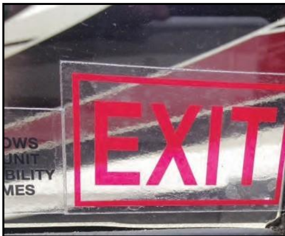
Figure 2-5: Emergency Exit Window
