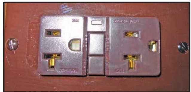
Figure 9-9: GFCI Receptacle
