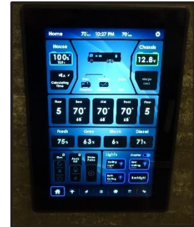
Figure 13-7: Water Pump Switch
