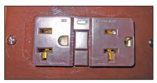
Figure 9-12: GFCI receptacle
