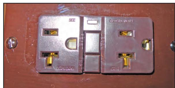
Figure 9-12: GFCI receptacle
